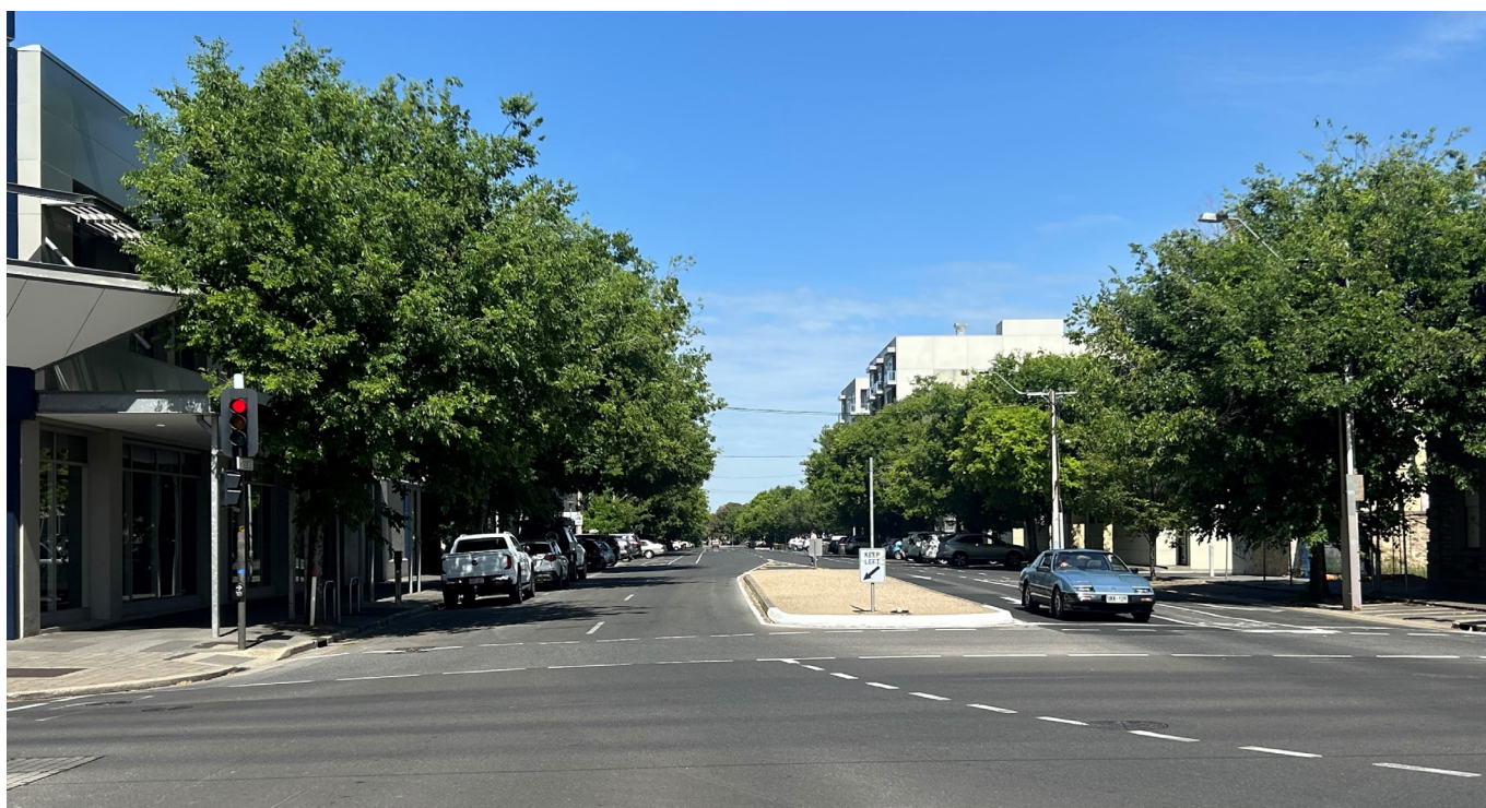
Sturt Street showing potential for new central median with trees from King William Street to Whitmore Square
