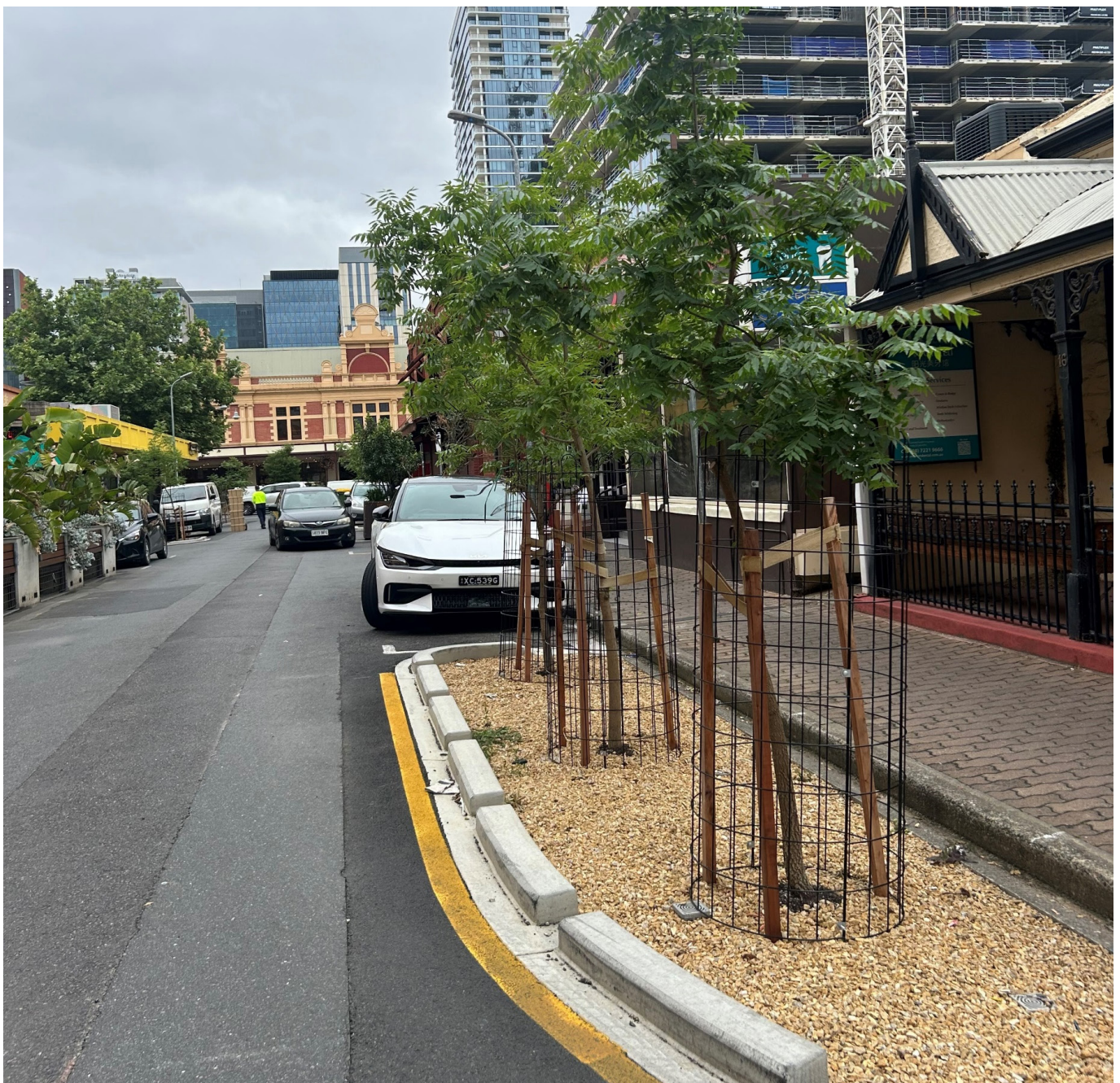
New tree planting along Market Street with WSUD, increased root zone under pavement and integration with street functions.
