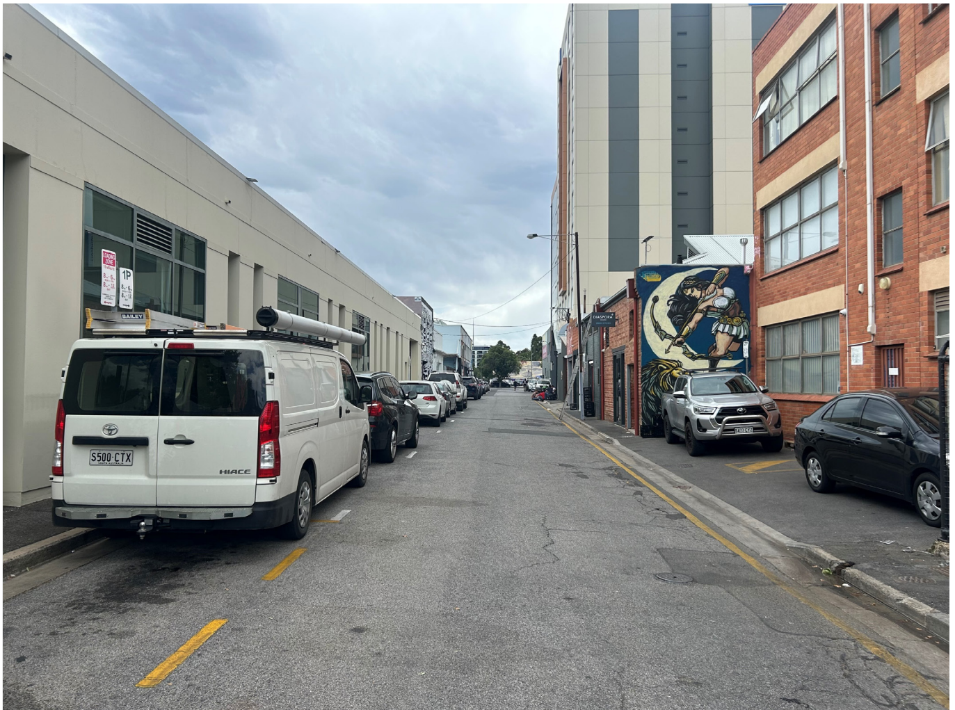
Gunson Street - a street with potential for greener outcomes, noting this may impact the availability of on-street parking
