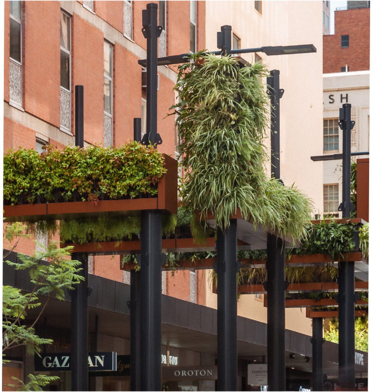
Example of arbour with vertical greening modules in Gawler Place
