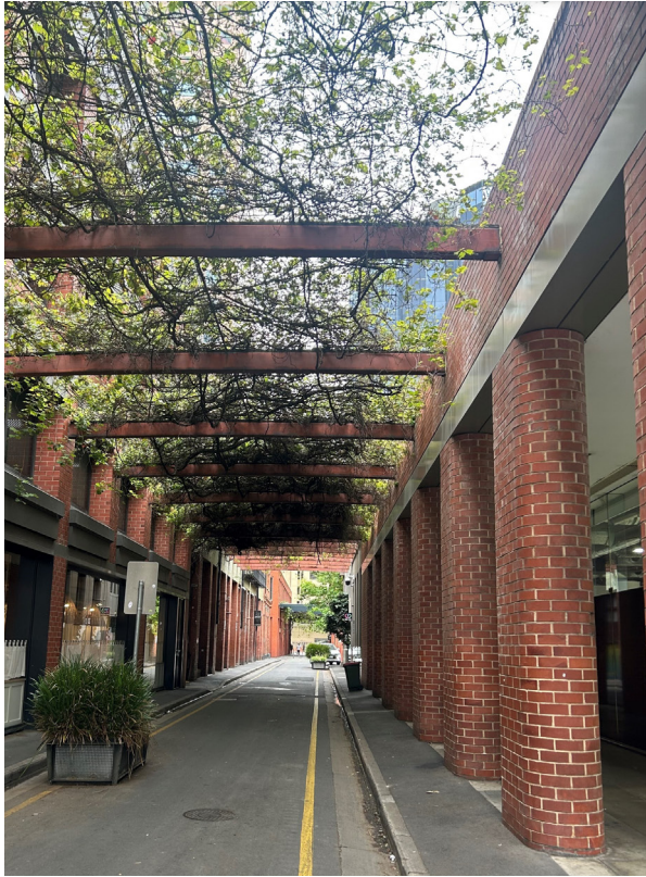
Example of arbour structure in Chesser Street
